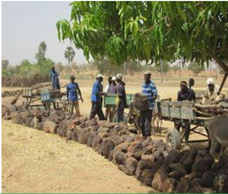
Source: Caritas Mali -Photos N ° 1 and 2: Realization of anti-erosion works / stony cords
